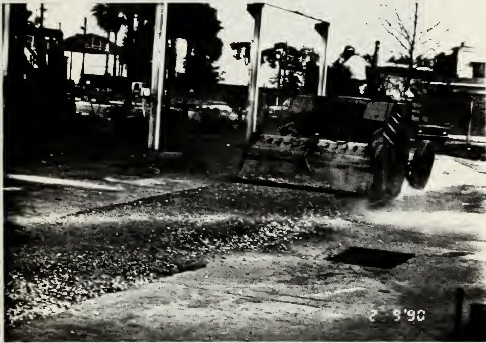
Figure 2.12 Dry Mixing of Aggregate and Cement Powder
